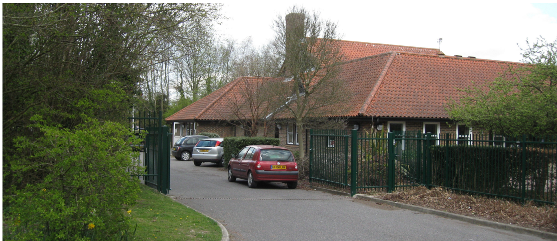
2. Section of the recently installed fencing under permitted development
